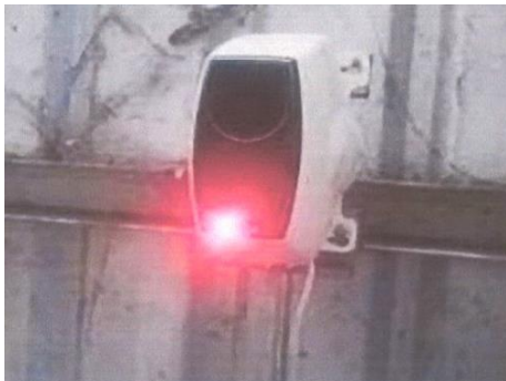
Smoke Beam Detector
